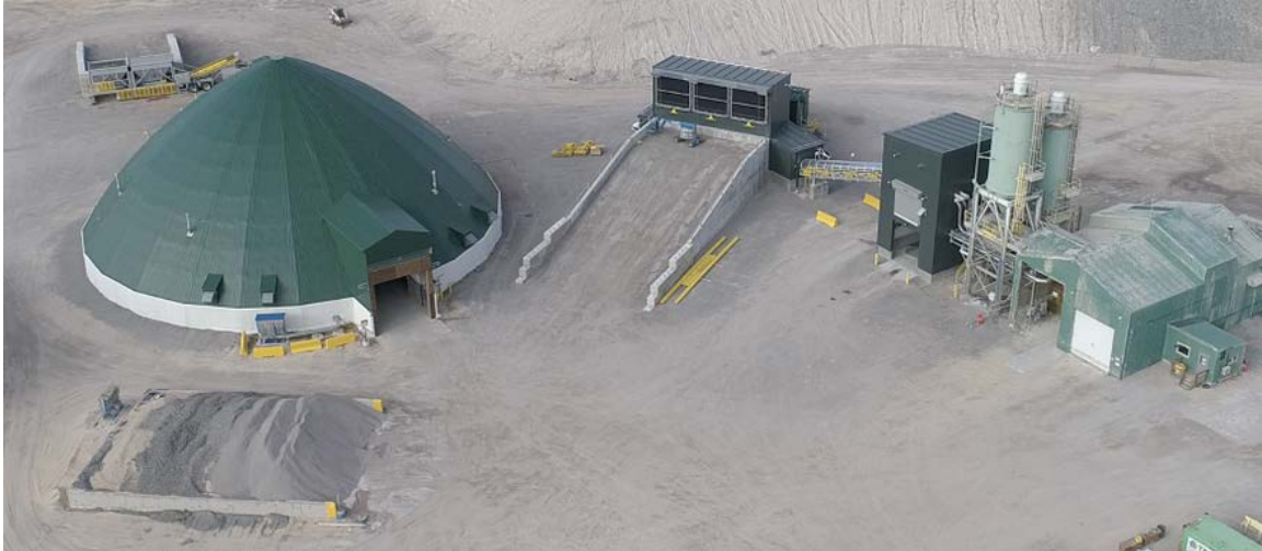
Figure 3.6-2: McArthur River concrete batch plant.
